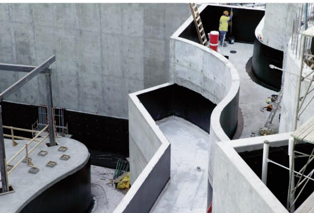
Many guest suites — such as those above with balconies — contained pools, spas, and planters. Coatings professionals literally used miles of Carlisle CCW MiraDRI 860 Sheet Membrane, a self-adhering product comprising 56 mils of rubberized asphalt laminated to a 4-mil polyethylene backing. Installation with roller, brush, or spray equipment typically began 7 to 14 days after the concrete was poured to allow time for curing. Field testing ensured nothing leaked above the casino or anywhere else.
