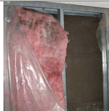
Fiberglass Batts: Steel studs are bridging insulation. Batts are also wet from trapped condensation.
