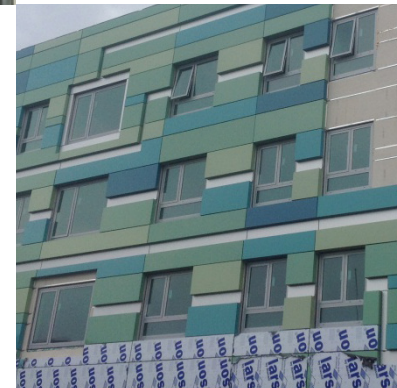
Polyiso foam board: Insulation is bridged with steel Z channels for attaching exterior panels.
